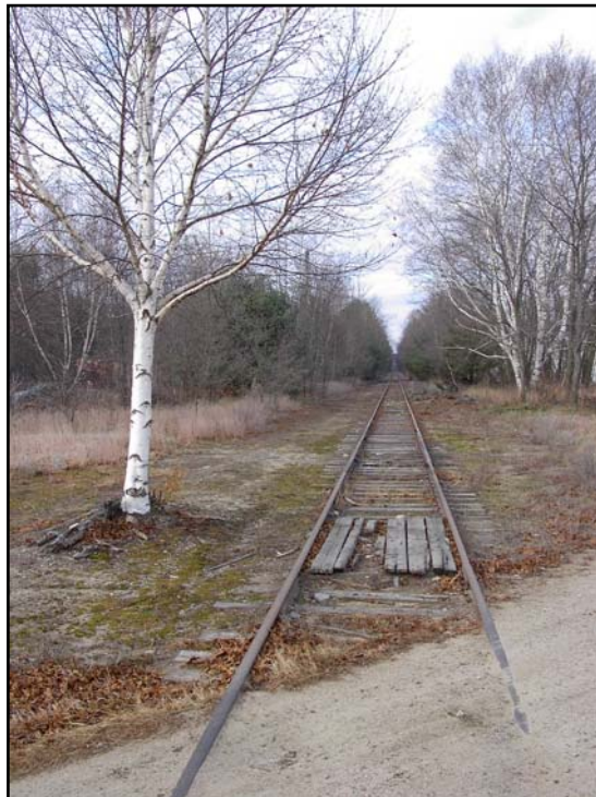
For parts of the line such as this one at Fair Street in Fryeburg, ballast is virtually nonexistent and ties are rotting
