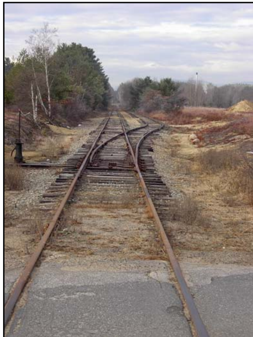
Sidings such as this one in downtown Fryeburg can be used as Team Tracks
